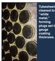
cleaned to "white metal," forming plugs set to gauge coating thickness.
